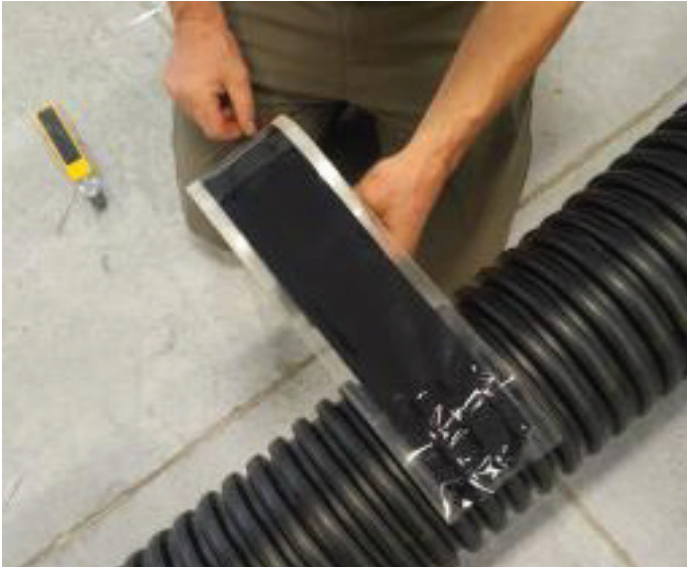
Figure 4-11: Seal pipe with black tape
