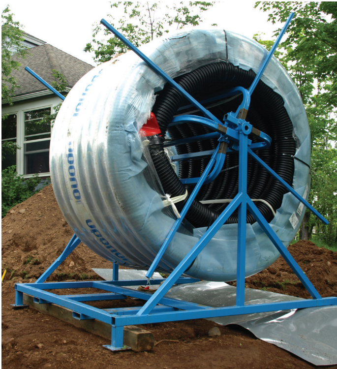
Figure 4-4: Stationary uncoiler
