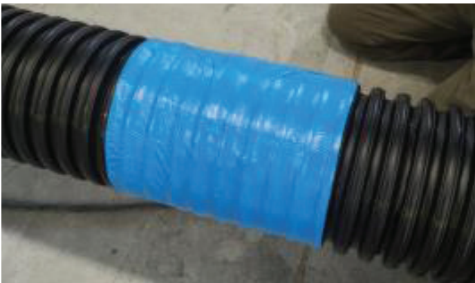
Figure 4-12: Seal pipe with blue tape
