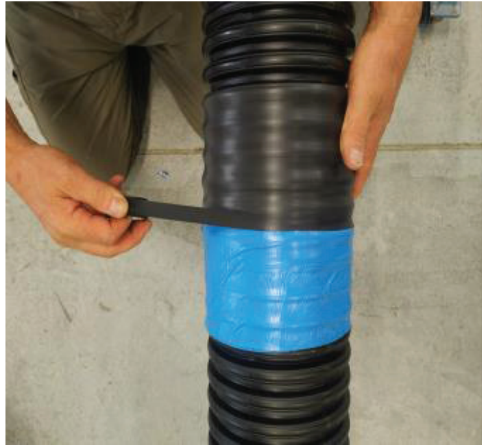
Figure 4-13: Seal with black outer tape
